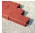
The use of clay pavers for streets, places, paths and gardens is as old as building itself. In order to permit the unhindered drainage of water as well as permanent evenness and full loading, a corresponding paving bed is necessary.
