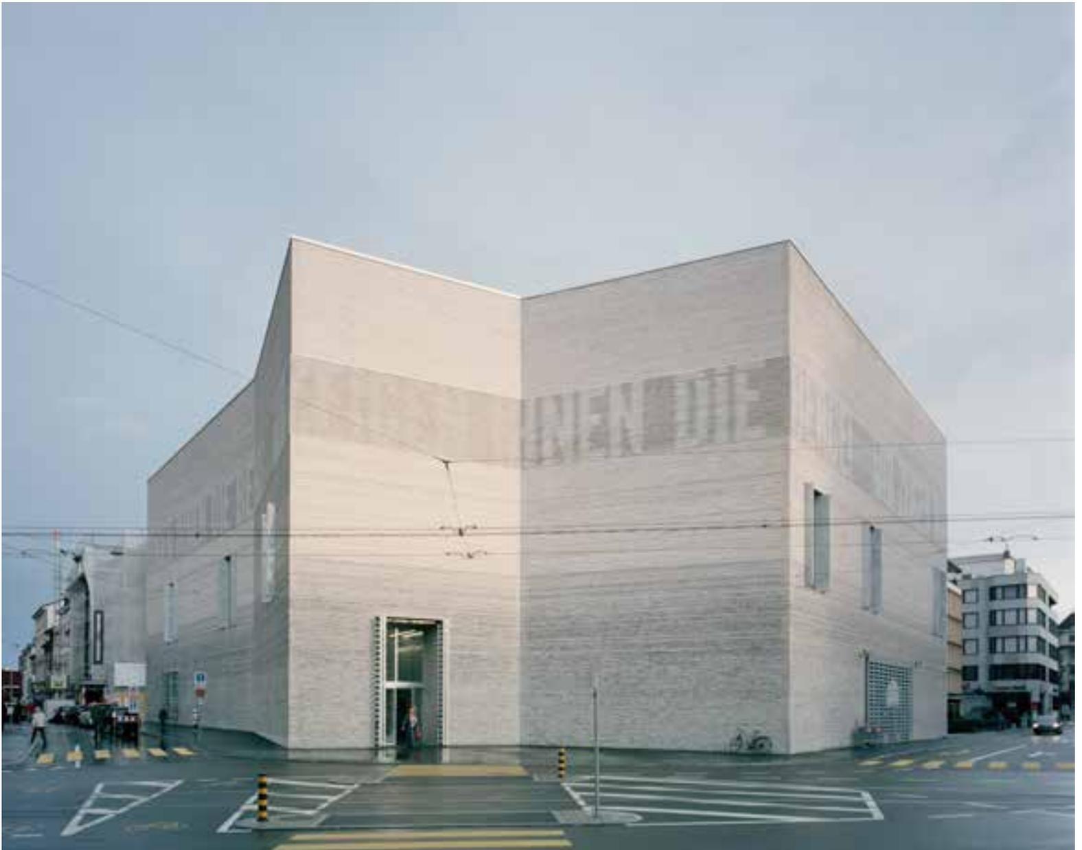
LEDs that send messages out into the urban space are integrated into the dark stripe.
