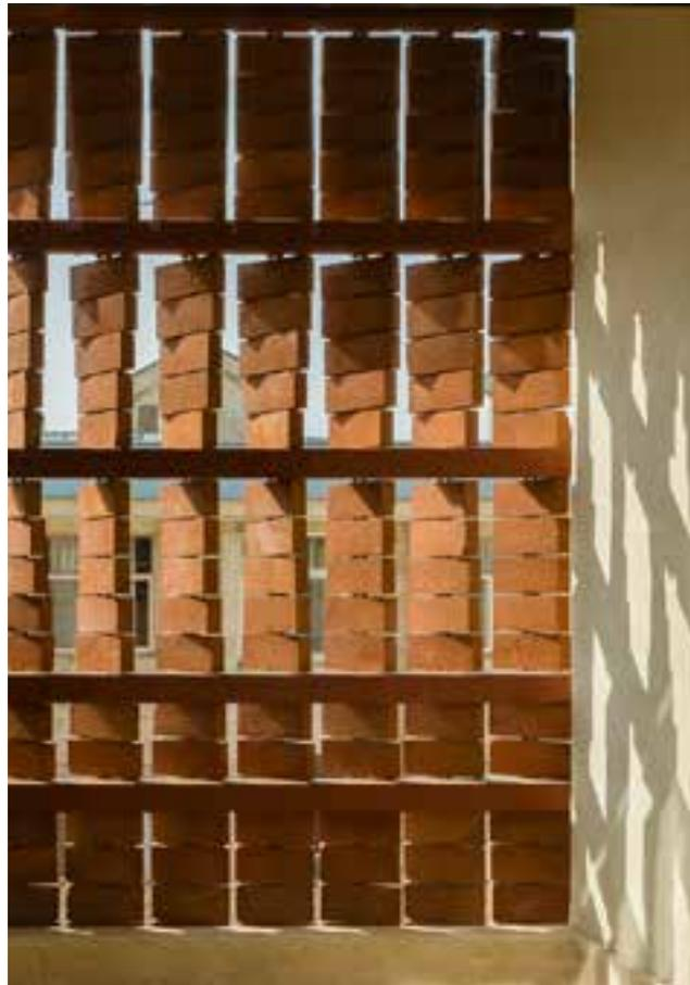
The bricks are not walled up, but rather placed on rods.
