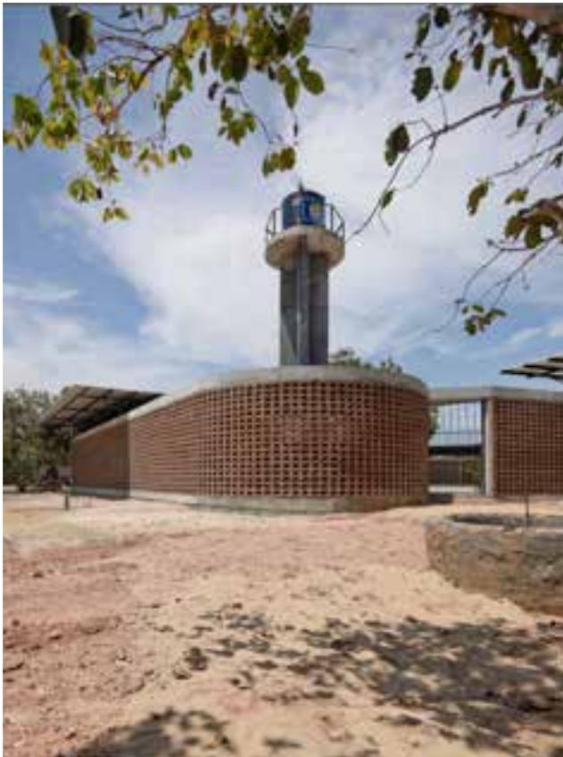
The bricks were produced on-site; the house was erected with the help of its users.
