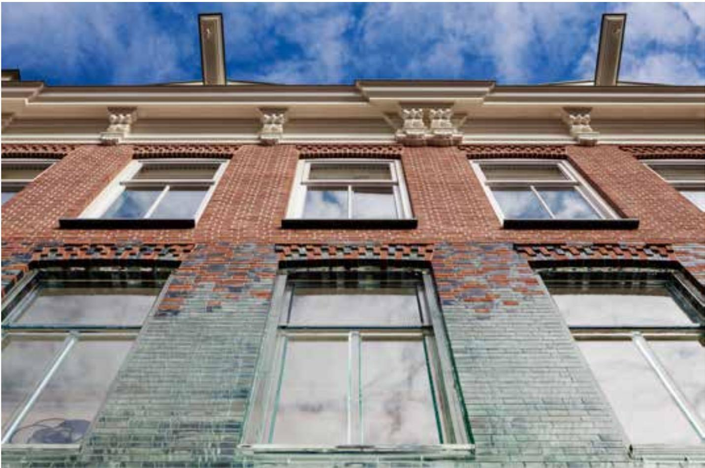
At the height of the first floor the glass bricks transition into fired bricks.
