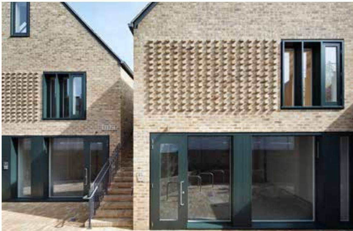
Bricks rotating out of the façade at a 90-degree angle structure the surfaces.
