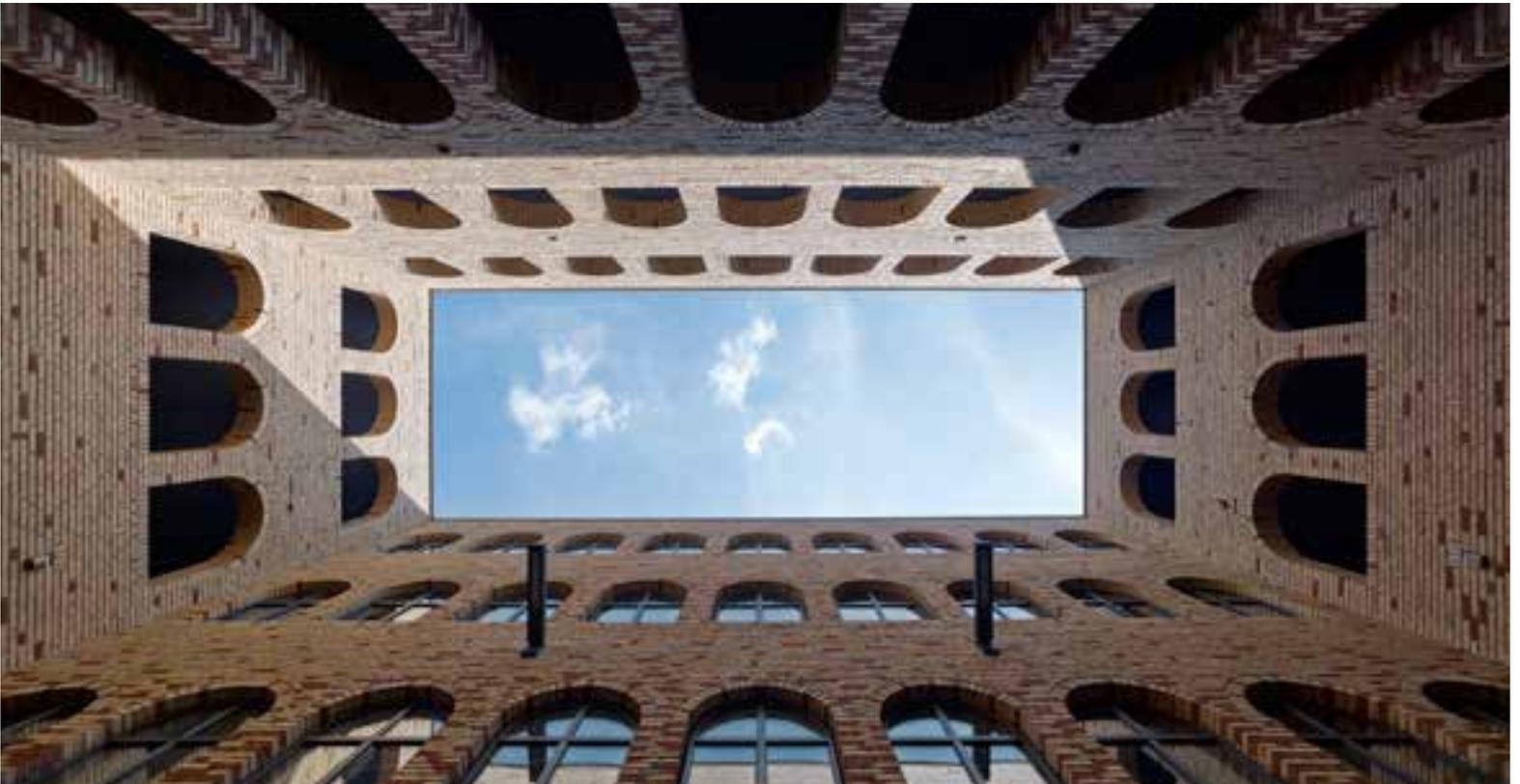
The round arches result from the constructive possibilities of the brick.
