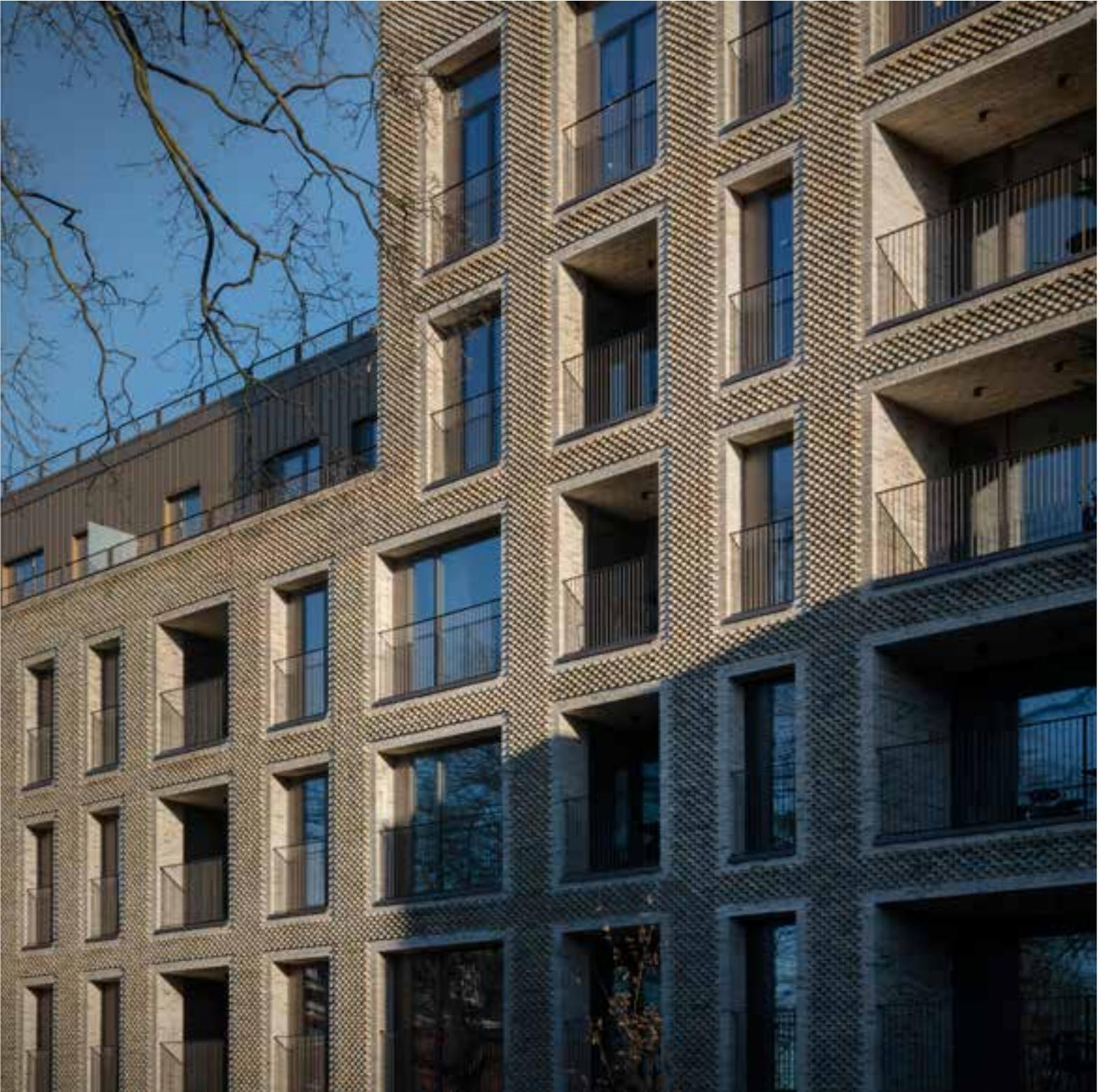
Bricks laid in a 45-degree, rotated bond result in a lively façade ornamentation.
