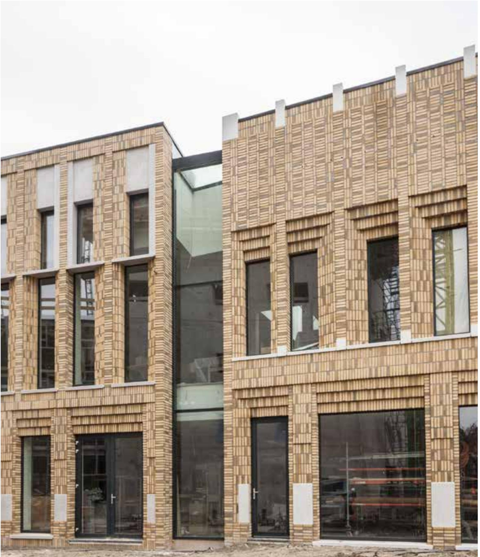
The entire façade is built out of prefabricated brick elements.
