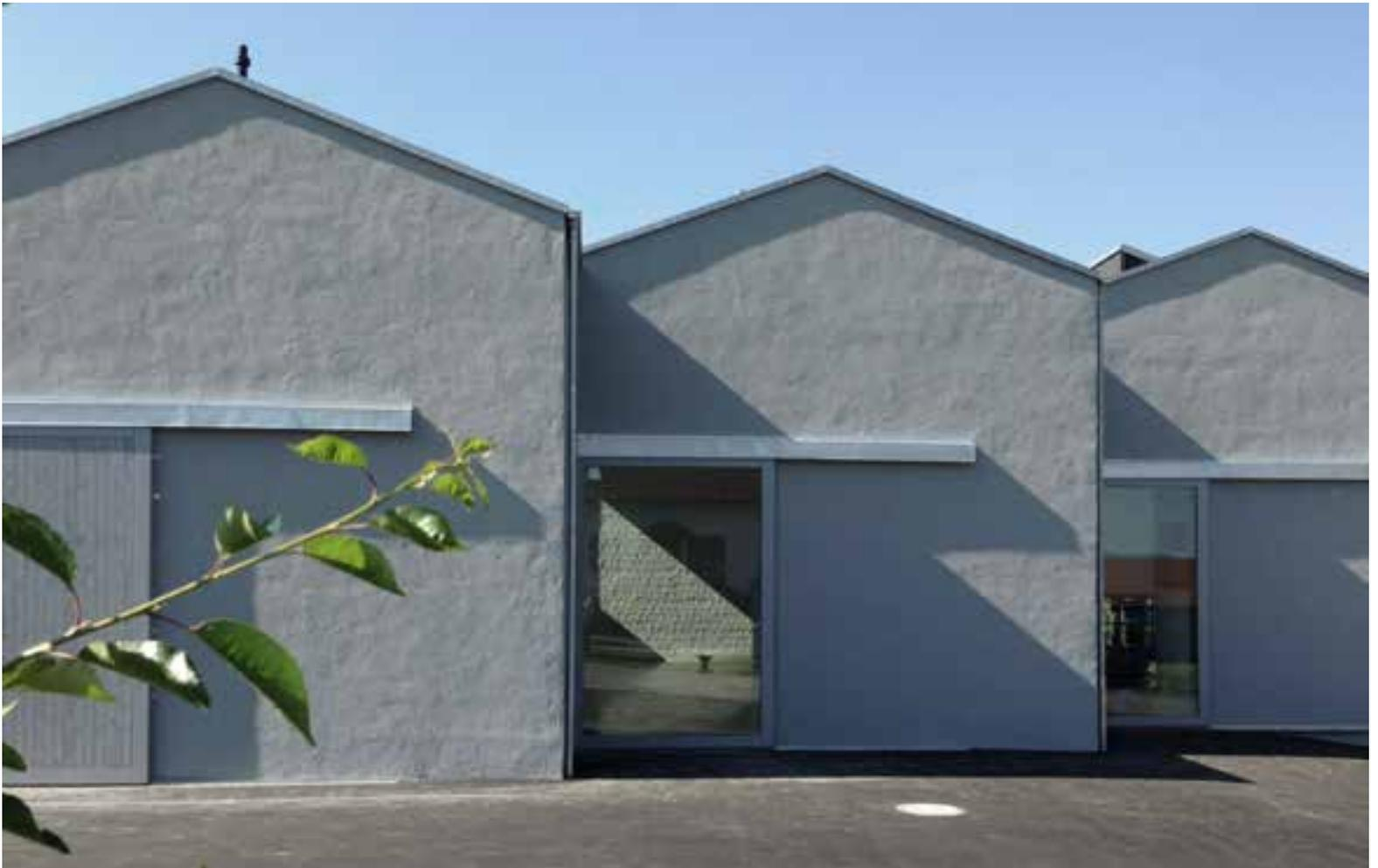
As simple as possible: brick masonry with a rough, bright plaster
