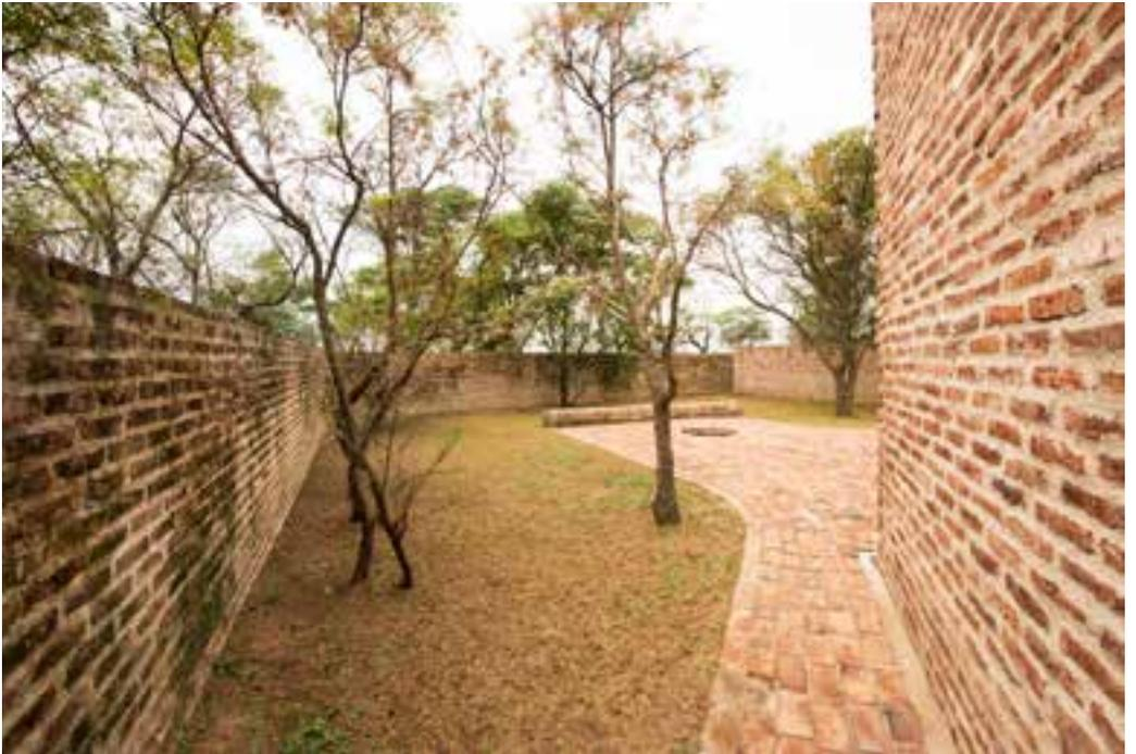
Old bricks were used for the external walls and the wall around the chapel.
