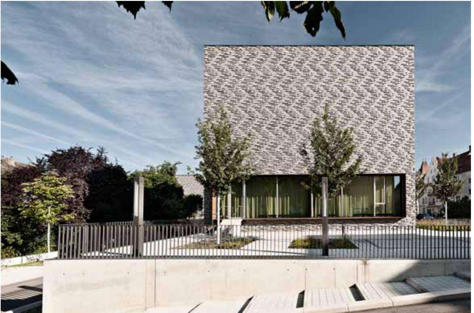
A fishbone structure emerges through the change in chromaticity, size and laying depth of the bricks.
