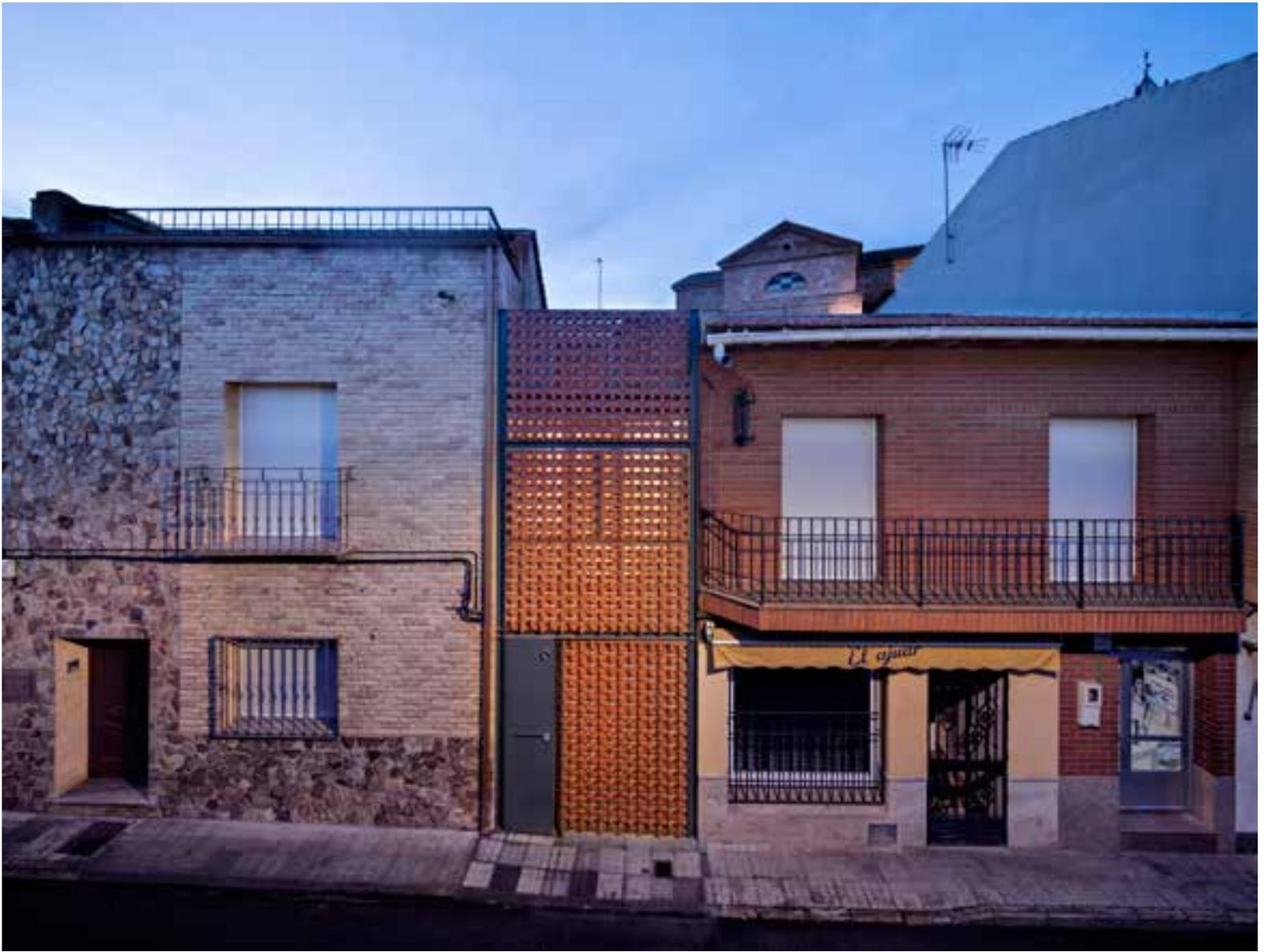
The ornamental-like structure of the façade is the result of bricks arranged vertically and edgewise, as well as rotated at a 90-degree angle.
