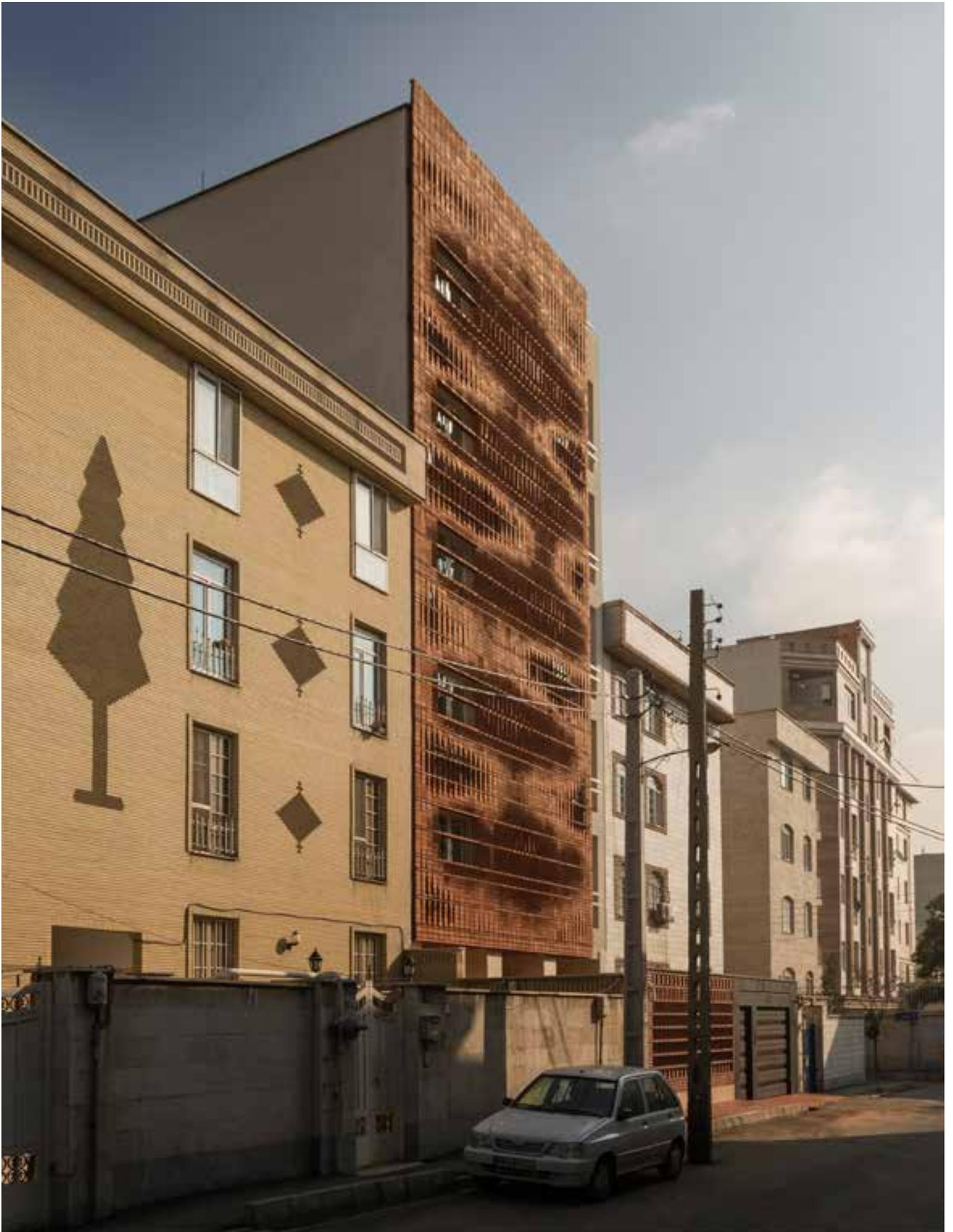
Depending on the function behind it, the individual bricks rotate more or less strongly out of the façade plane.
