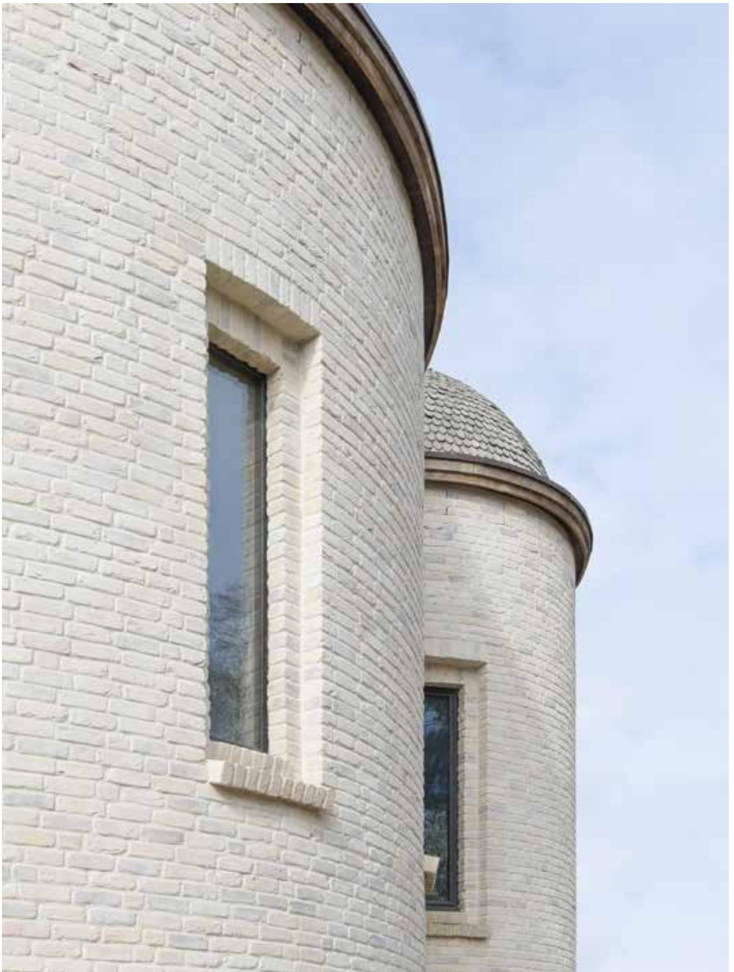
Hand-molded bricks covered with white slurry allow the original color of the bricks to shimmer through.
