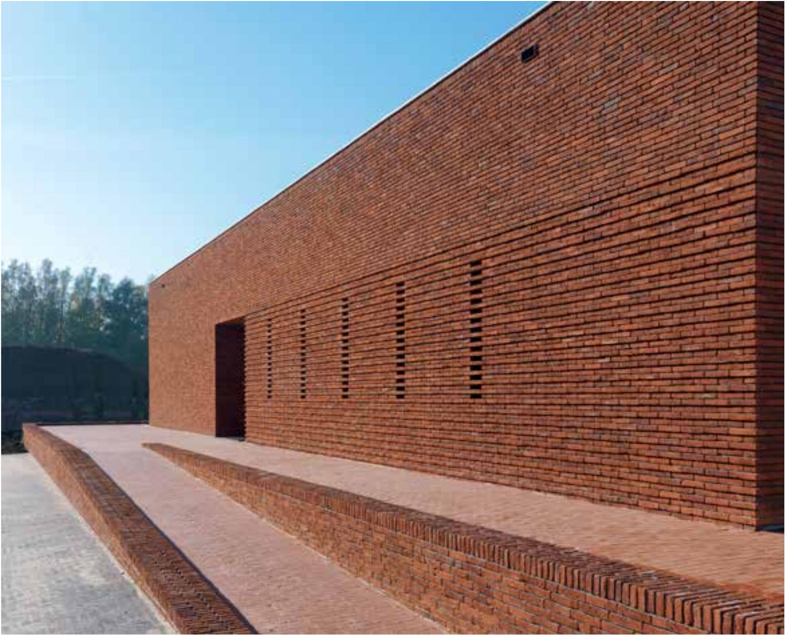
The brick is produced on-site and bricked up with deeply recessed bed joints and without butt joints.
