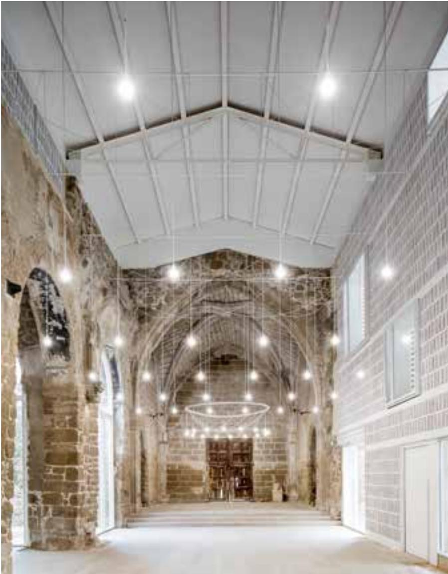
A gabled roof with an open soffit connects the old and the new.
