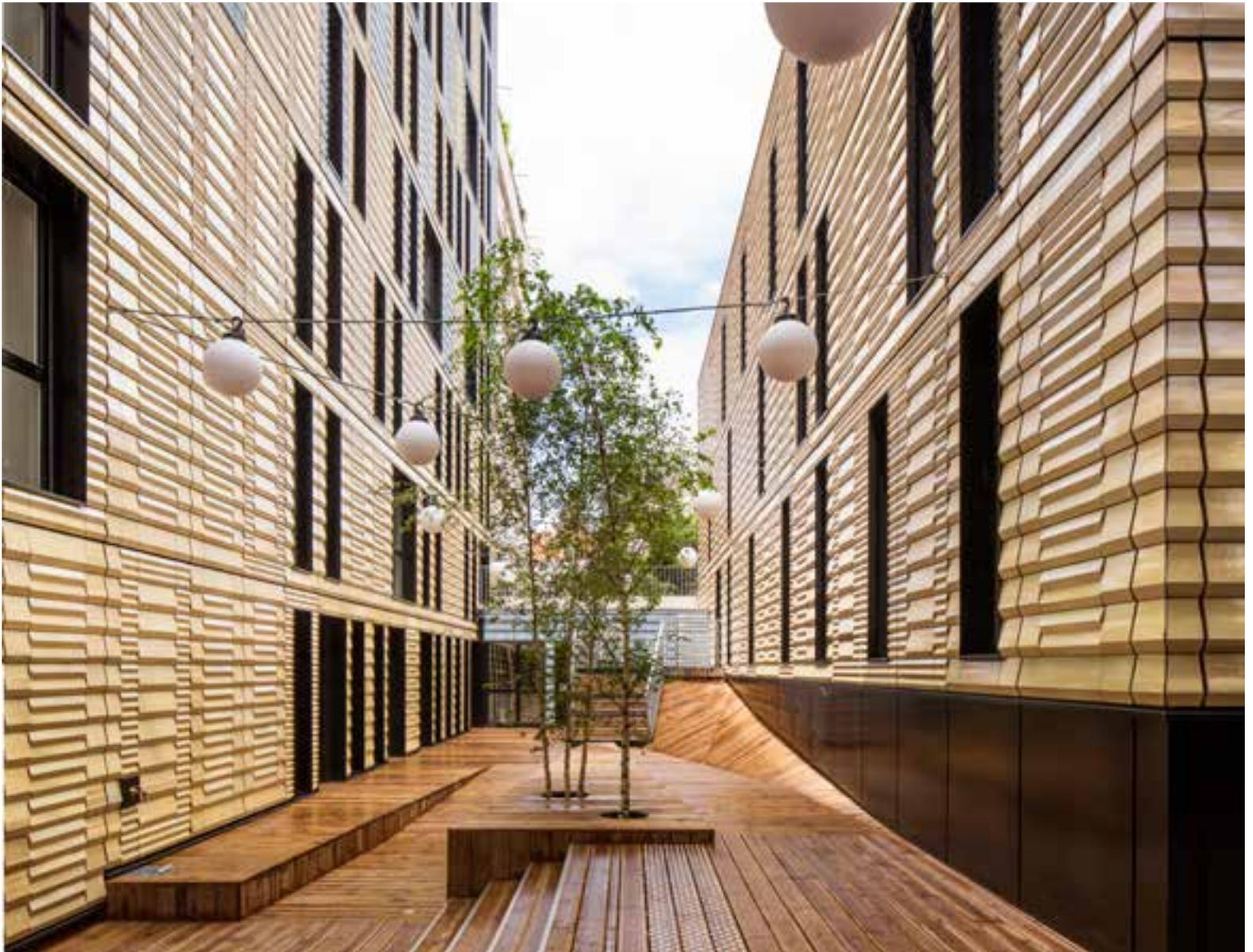
Three different 45 × 45 cm 3D-tiles are the basic elements of the façade.
