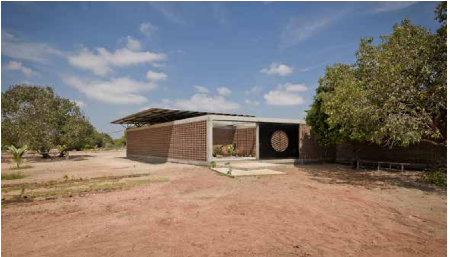
In order to guarantee good ventilation, large sections of the brick masonry were laid in an open bond.
