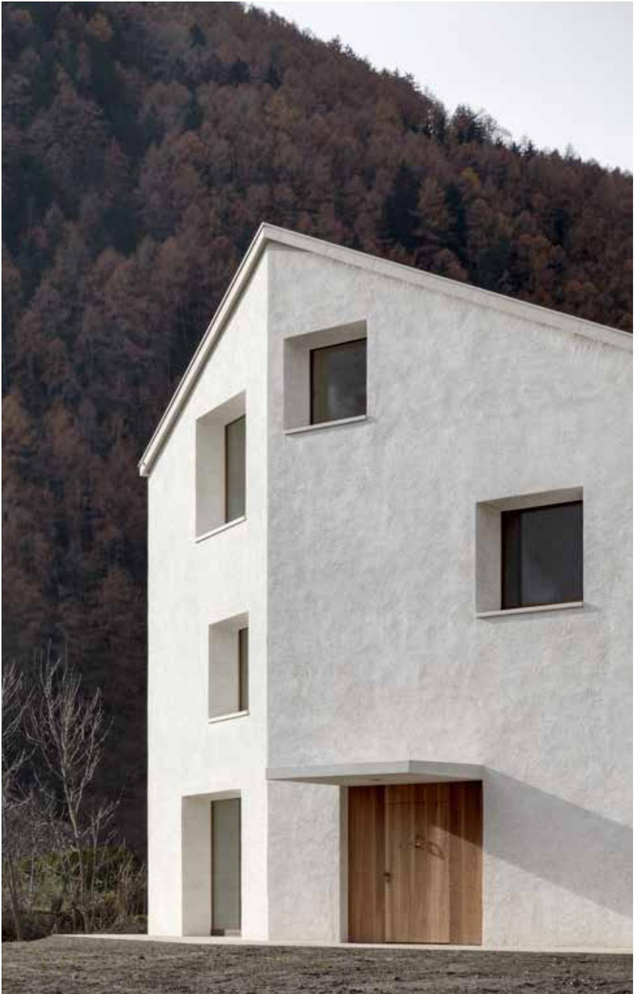
The brick masonry was rendered with a plaster made of lime, white cement and local sands.
