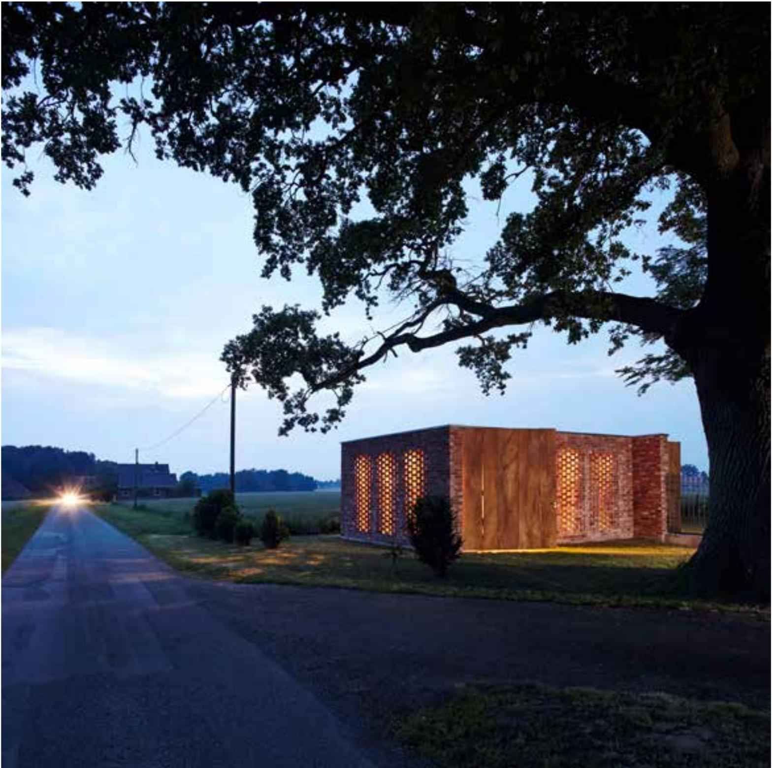
The perforated façade ends where the load-bearing pillars stand.
