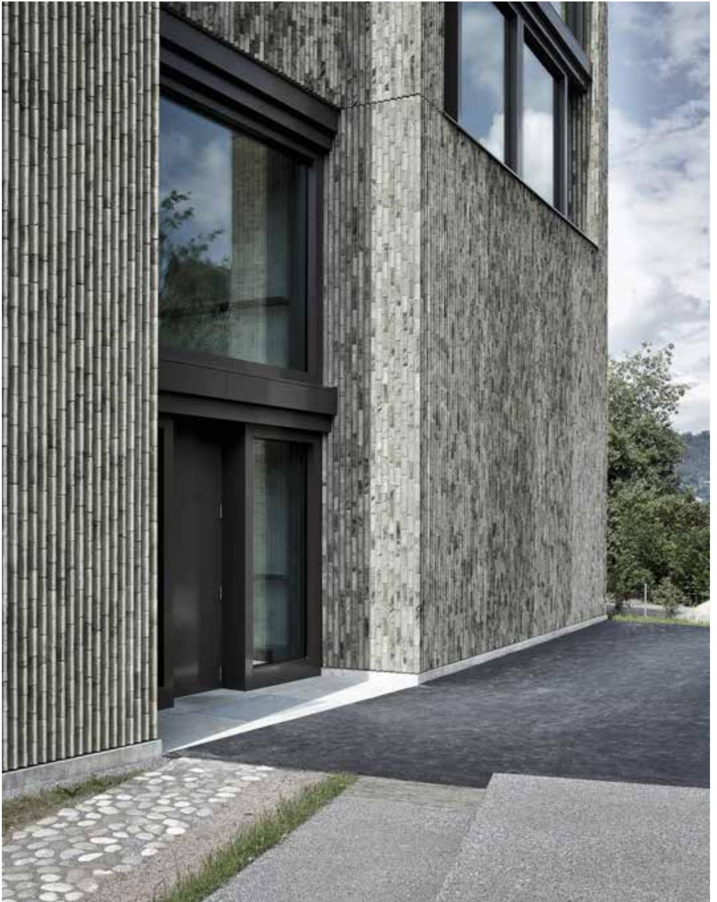
Framing elements with vertically laid bricks were mounted onto the façade.
