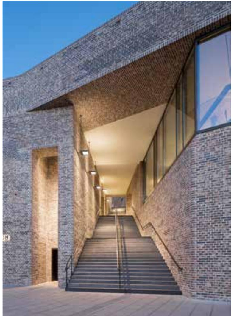
The color gradient of the bricks gets darker going upwards while the joints get deeper.
