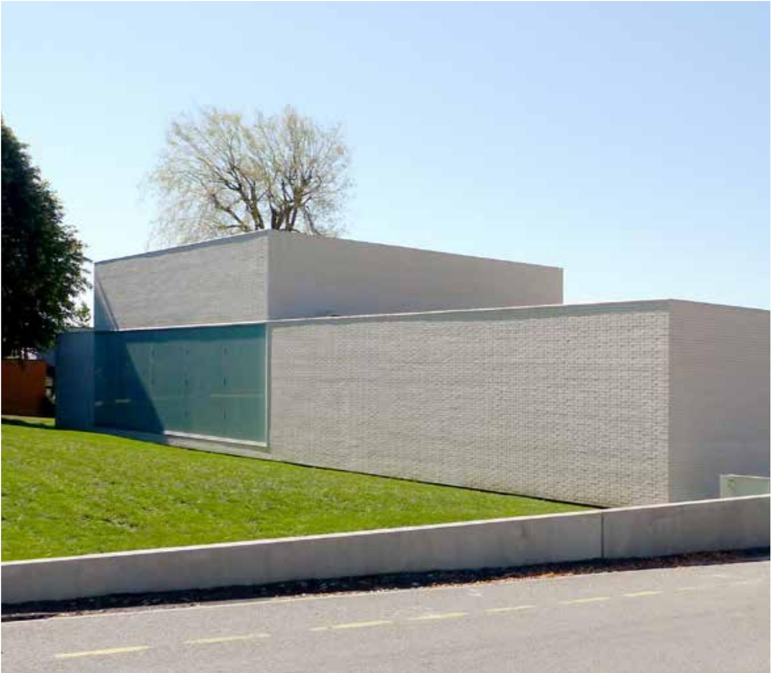
Exposed concrete and white clinkers with gray joints on the façade
