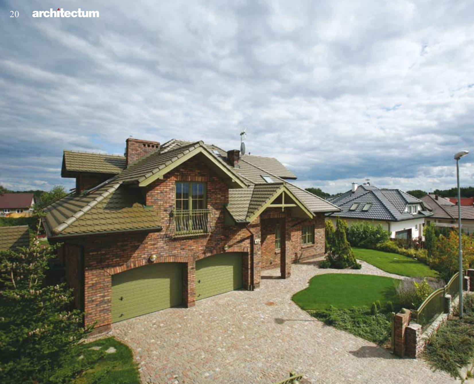
The olive-brown façade bricks harmonise perfectly with the imposing roof of green engobed beaver tiles.
