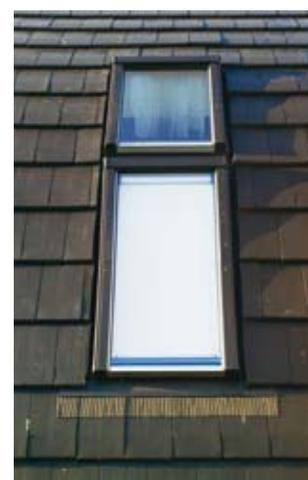
For the roof covering of his single-family house built to ecological standards, the architect chose anthracite-coloured matt clay roof tiles, which are inexpensive and simple to lay.
